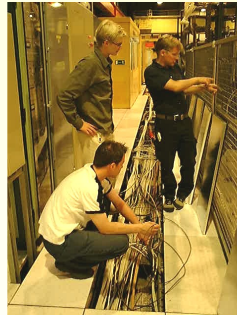
Picture 3: HIP students installing cables for SiBT at H2
