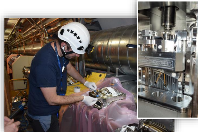
Inspection of TCPC by SY/STI
