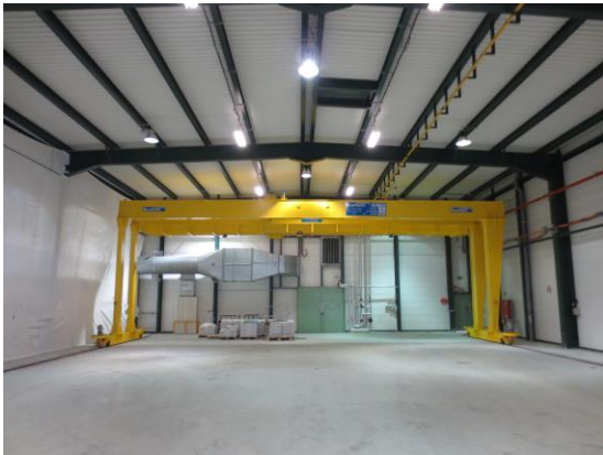
Installation of 5T gantry crane
