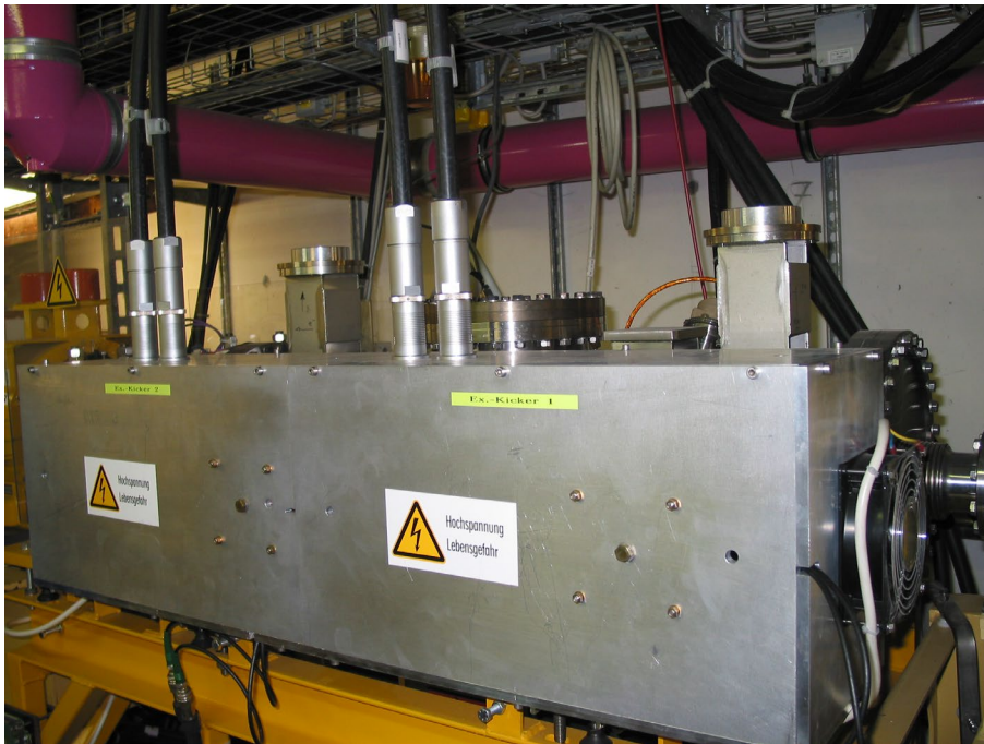
Two booster extraction kicker magnets
