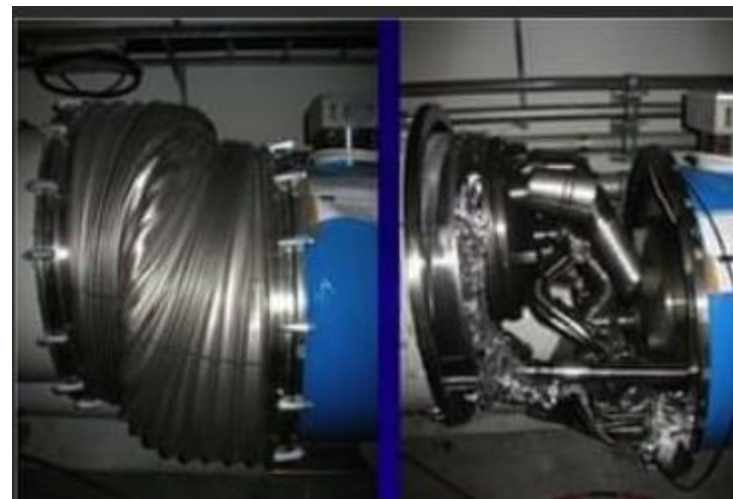
Joint failure damaged 50 magnet
