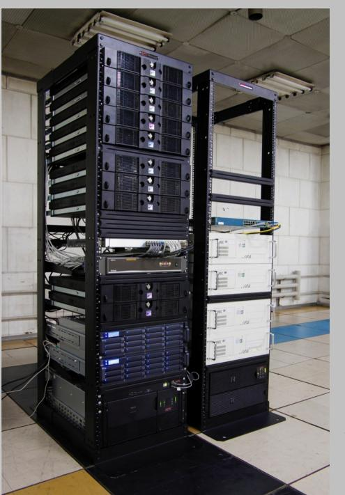
WNs (40 CPU cores, 200 GB RAM, 5TB on local HDDs) Cisco Catalyst 3750E (24x1G + 2x10G)00 Axus Yotta B 10 TB Axus Yotta B 15 TB APC 2/2+1 ATS (16A)
