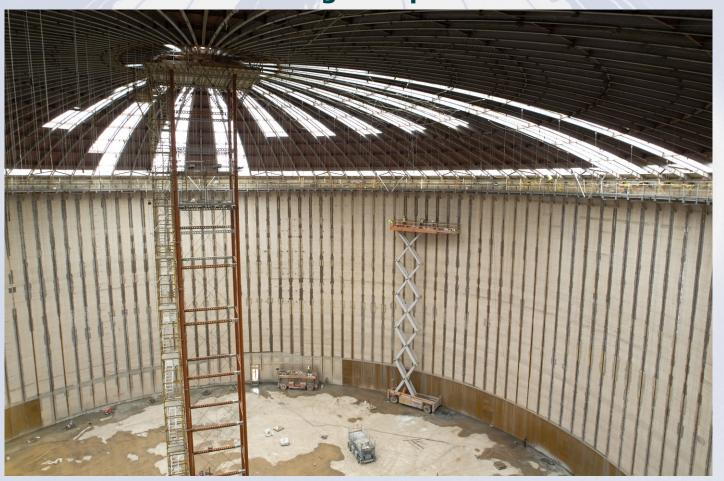
**Erecting and welding outer tank shell liner**
