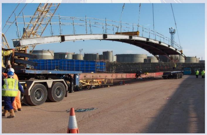
Roof construction - lifting petals into position
