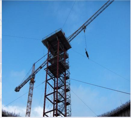
**Roof construction – transport petals from storage**
