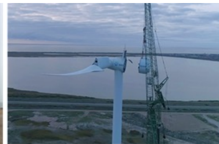
(left) The 3.6 MW EcoSwing HTS generator (blue, 4 m diameter) next to its conventional counterpart with the same power rating (red, 5.4 m diameter), prior to (right) its lift onto the turbine
