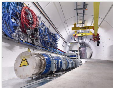
First phase of installation of FASER in the LHC tunnel
