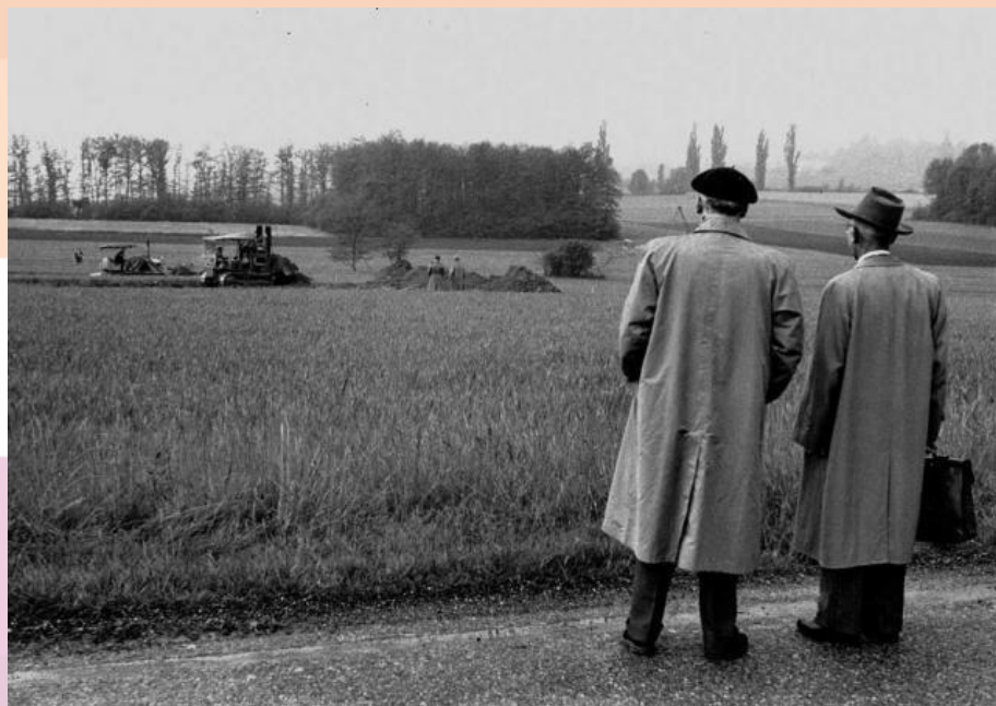
Groundbreaking at current CERN site in Meyrin, Switzerland, 1954.
