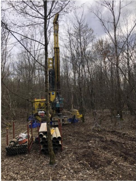
➤ Drilling machine in place
