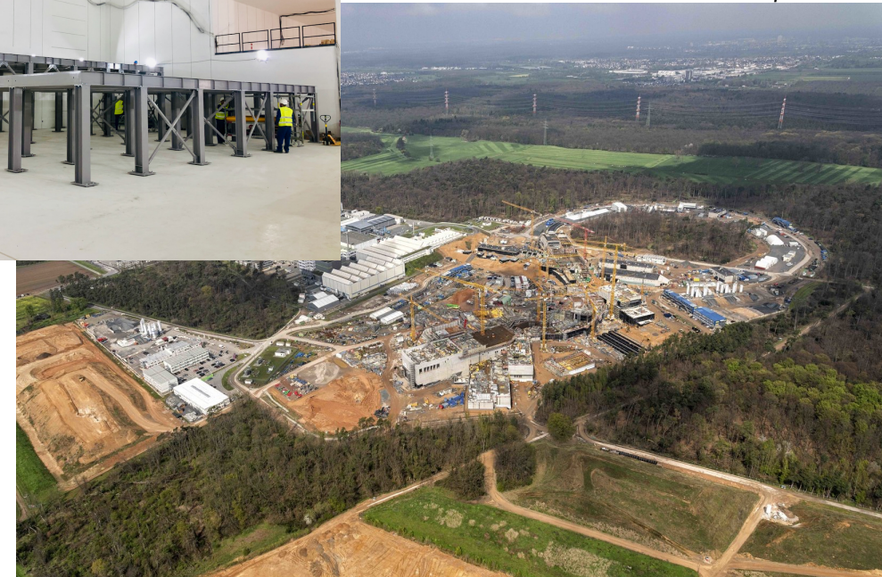
FAIR construction site (Darmstadt, Germany) Photo as of April 2023
