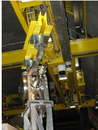
Target during installation TBID & remote lifting beam Horn with remote lifting cradles (in red)
