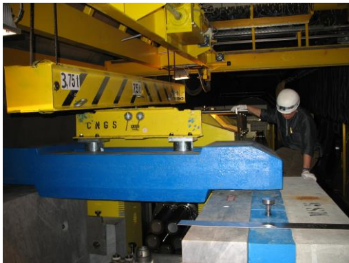
Remove roof shielding
