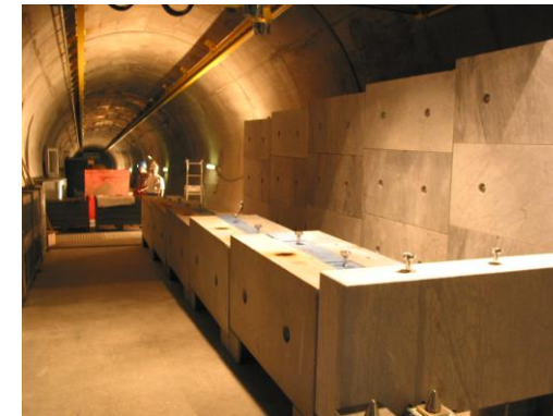
Remove all shielding blocks
