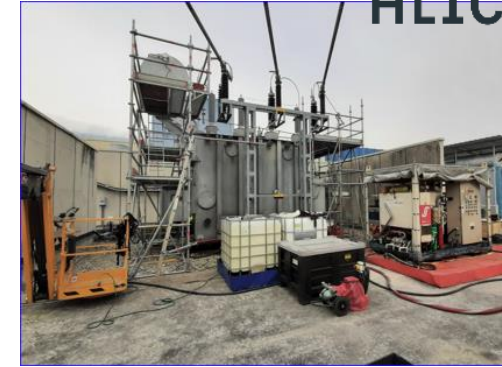
Maintenance on the 66kV transformer (EN-EL)
