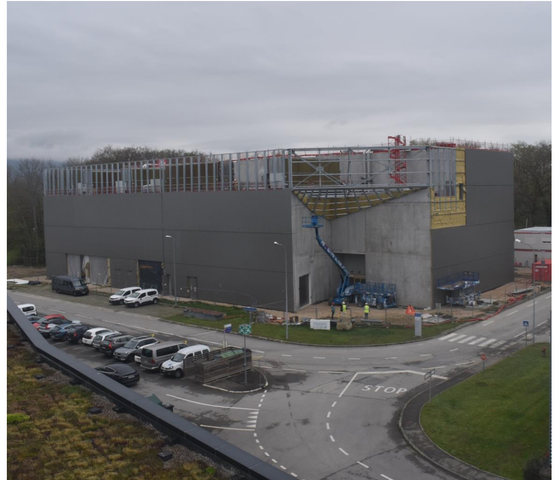
Exterior Finishings (Thu 20 th April)
