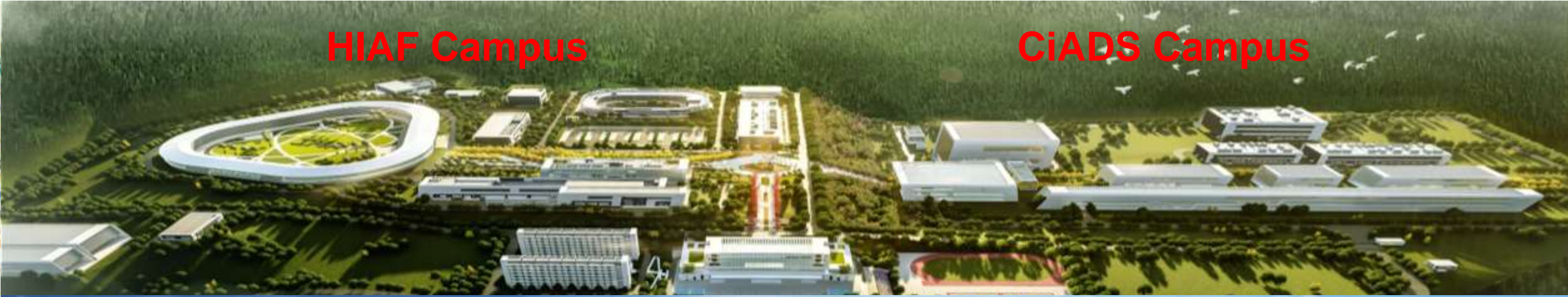
Civil construction (@June 2023)
