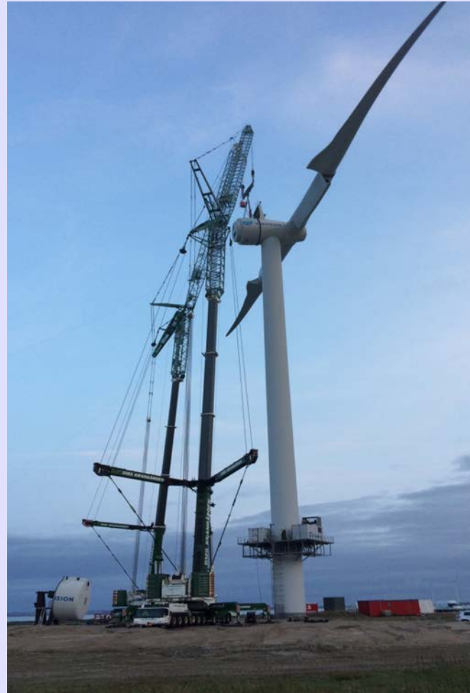
Lifting onto the Envision turbine
