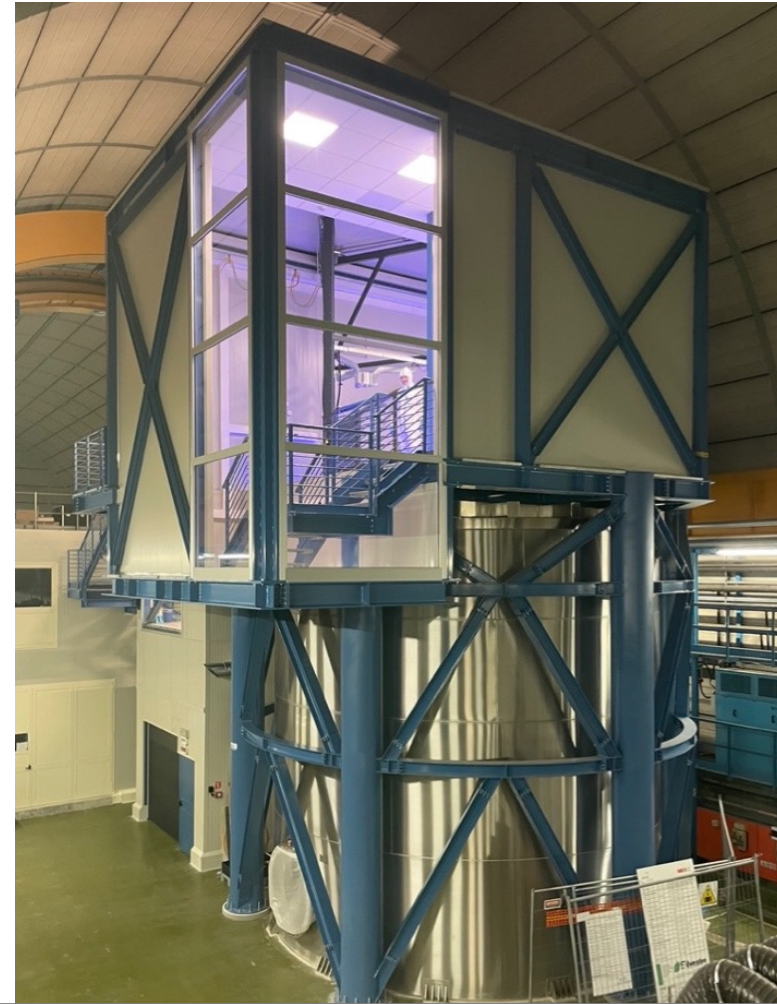
COSINUS facility completed in Aug, 2023
