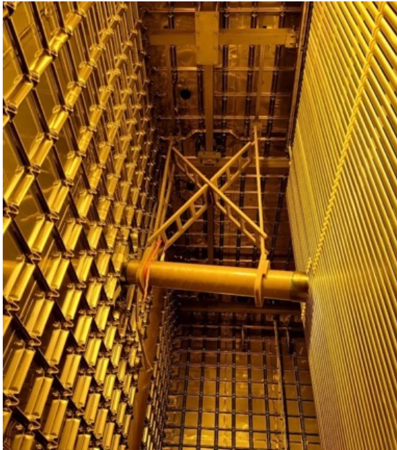
Installation of new, longer beam plug inside cryostat.
