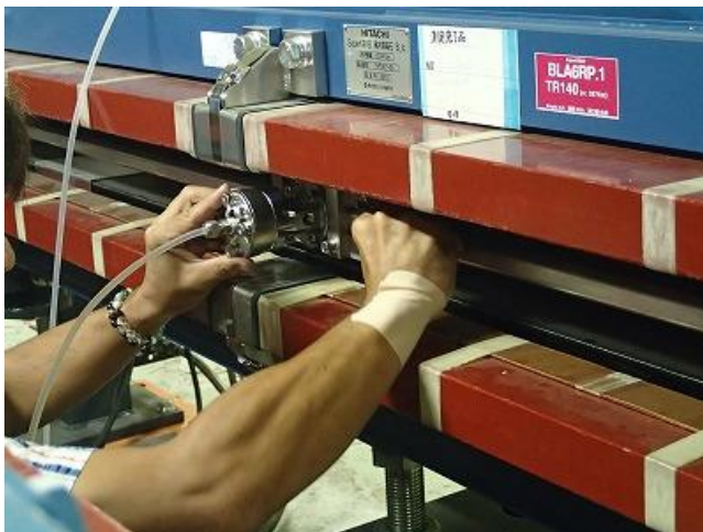
Knocking of beam pipes for bending magnets
