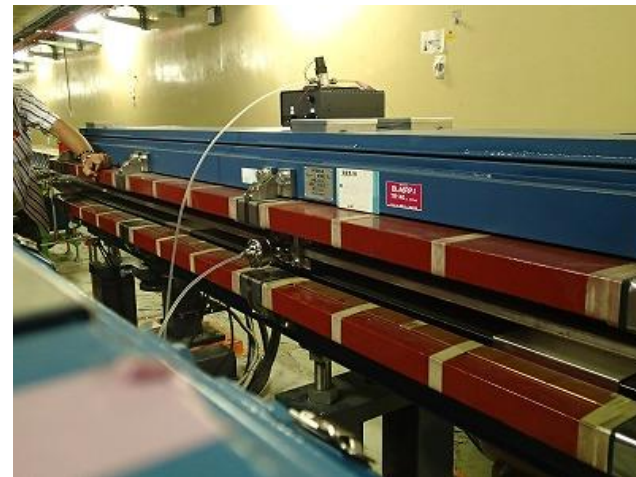
Knocking of beam pipes for bending magnets
