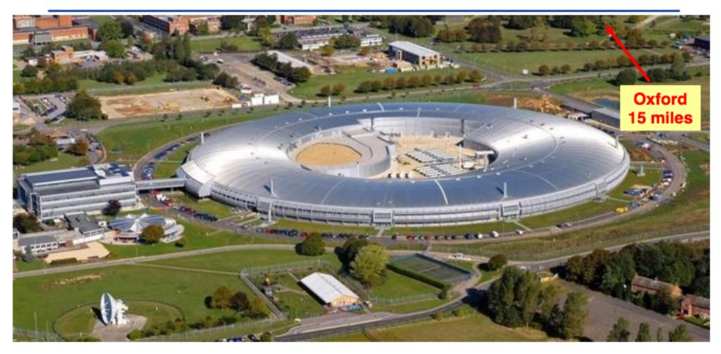
Diamond is a third generation light source open for users since January 2007 100 MeV LINAC; 3 GeV Booster; 3 GeV storage ring 2.7 nm emittance – 300 mA – 18 beamlines in operation (10 in-vacuum small gap IDs)
