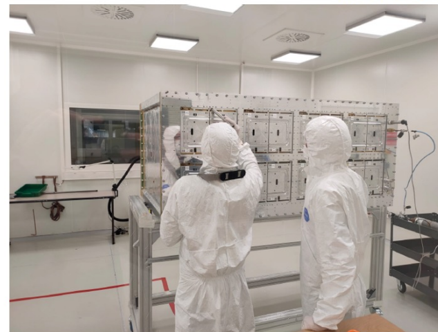
Leak test after ERAM installation
