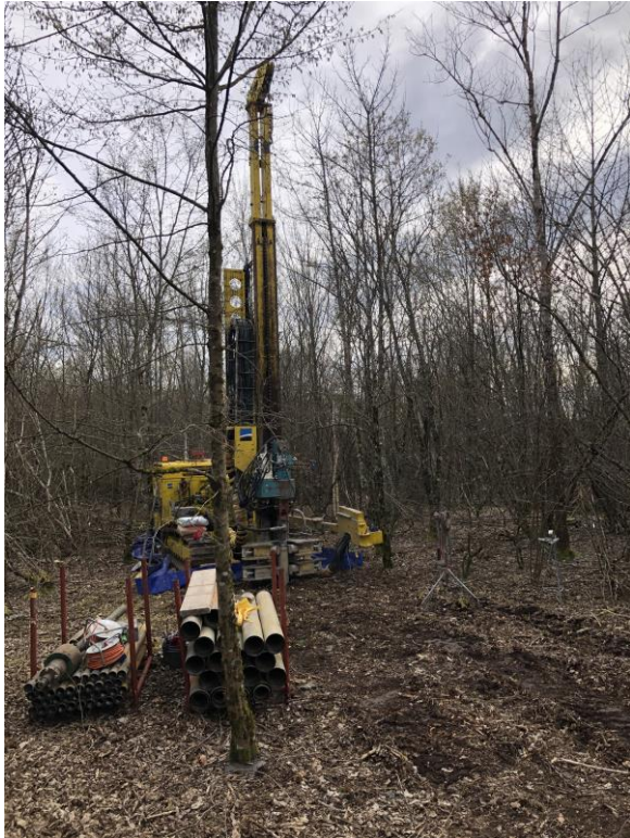
➤ Drilling machine in place
