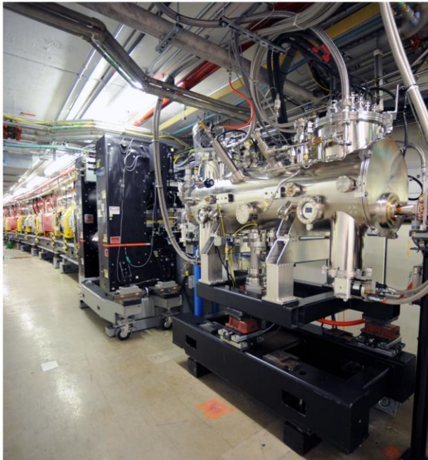
Helical SCU installed in APS
