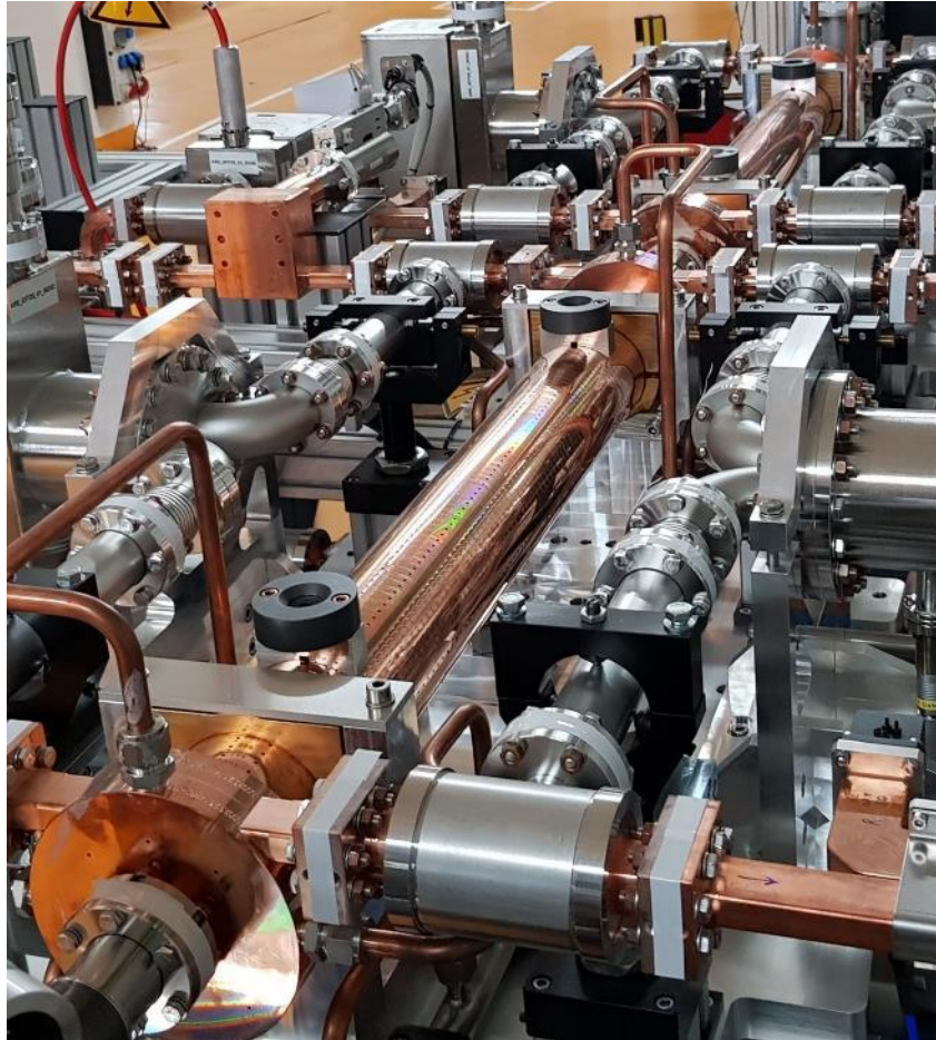
PolariX TDS installed at the ARES linac.
