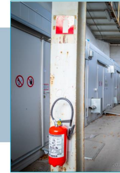
B. 128 (470m 2 ). Chemical containers.
