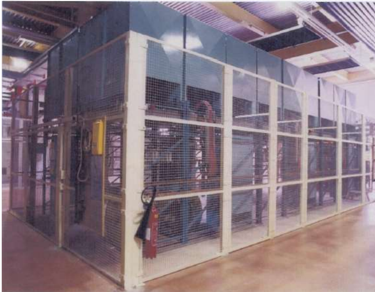
Stainless steel resistor bank of Tore Supra
