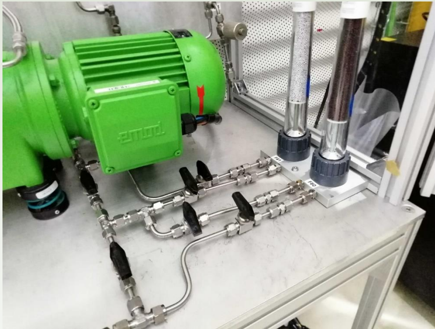
Filters in the gas system
