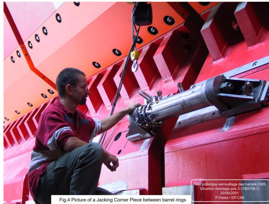
Fig.4 Picture of a Jacking Corner Piece between barrel rings
