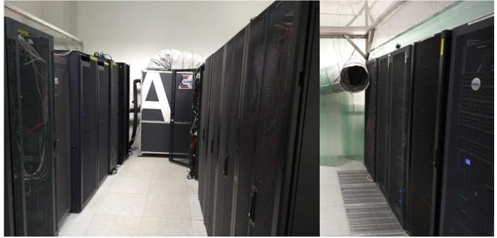
Pictures show the cold air directed into the cold aisles, (Originally directed under floor but insufficient pressure meant it stayed there)
