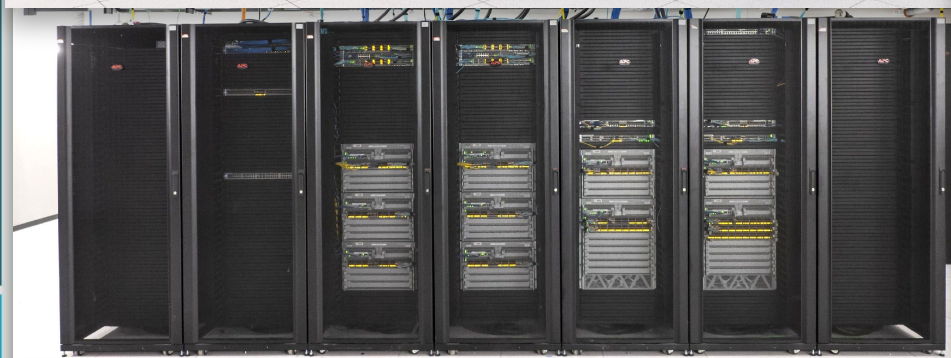
B725 Central Network Equipment Is Deployed & Active (10x 400 GbE ready Arista modular chassis with 48x line cards slots in total)
