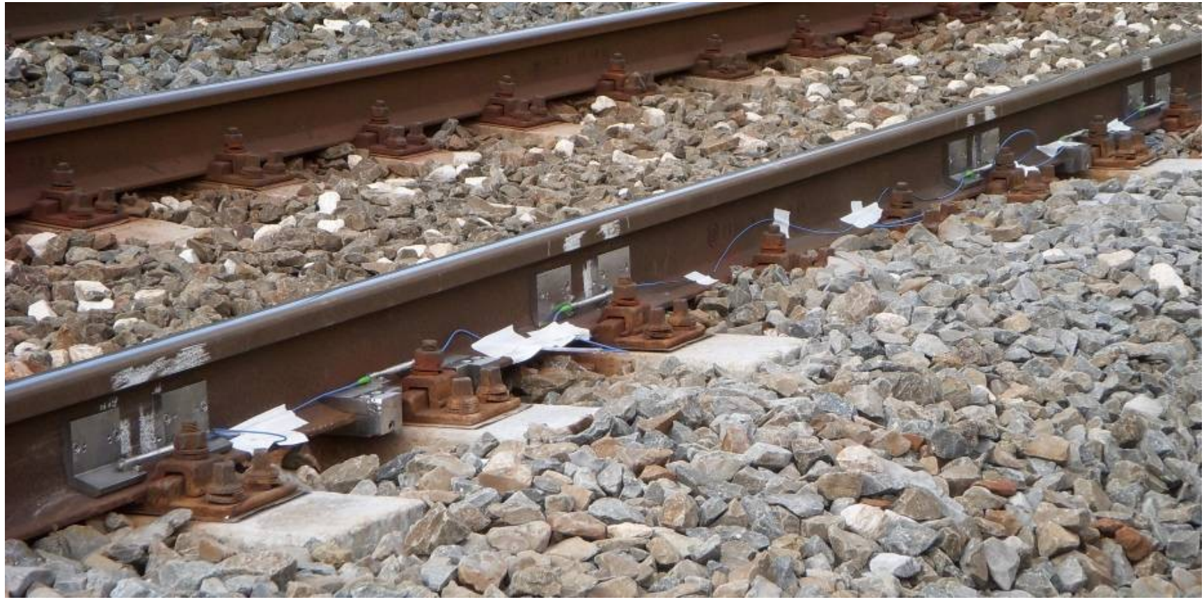
FBG packaged in mettalic holders along the railway
