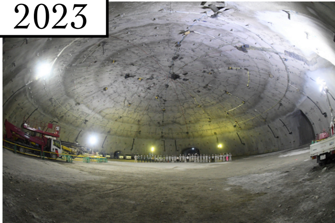
Cavern Dome Completed
