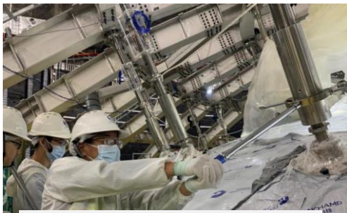
Supporting bar installation
