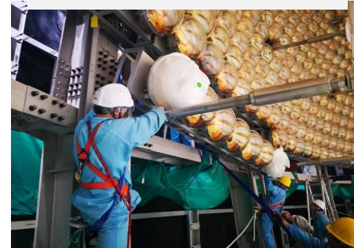
Installation of CD LPMT
