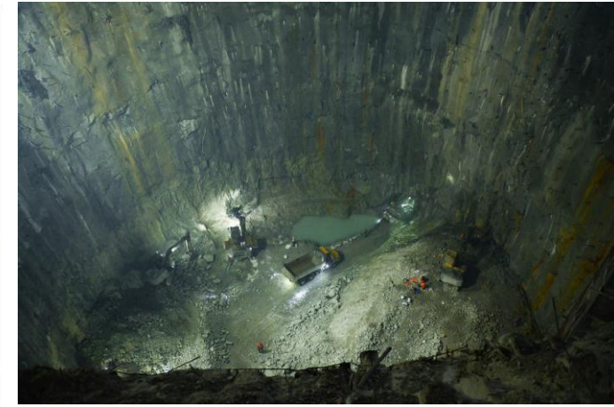
Cavern and water pool excavating
