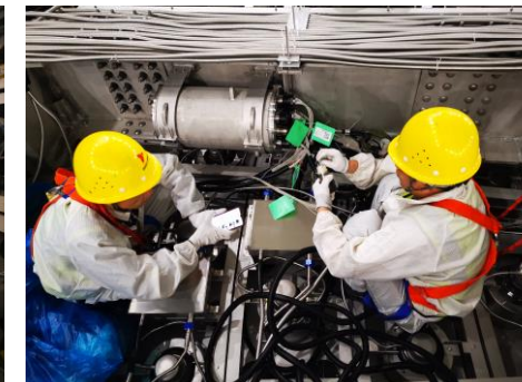
Installation of sPMT and electronics
