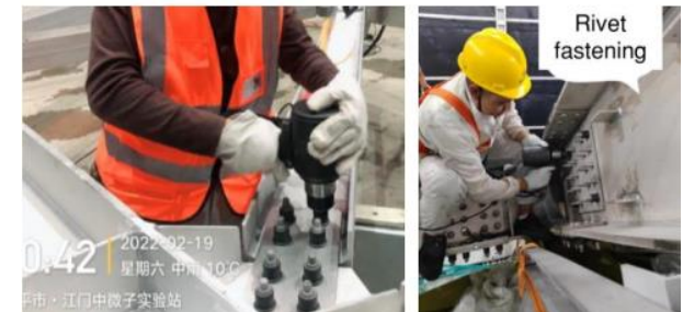
Bolts and riveting
