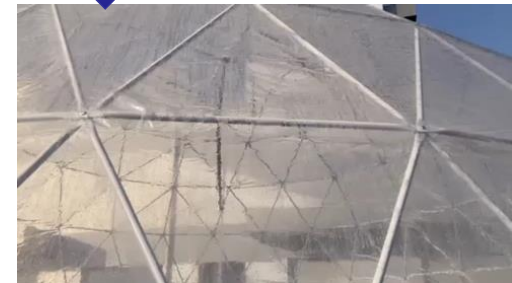
Prototype test for water spray cleaning
