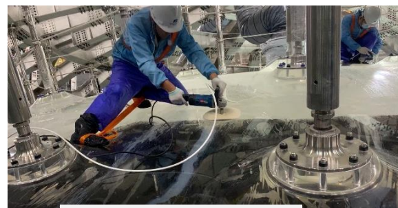
Bonding line sanding
