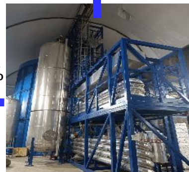
4) Gas stripping to remove Rn and O 2
