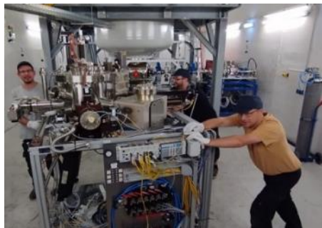
Dismantling of the PPF ( September 2023 )
