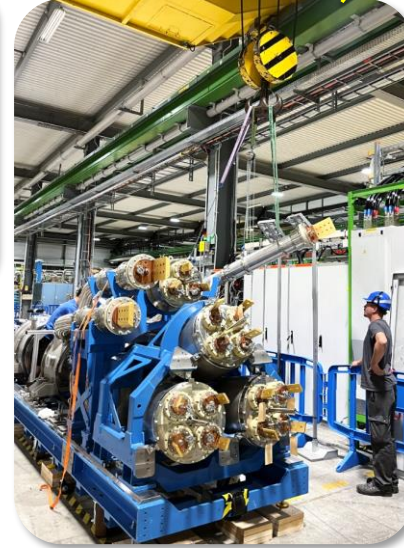
18kA current leads installation
