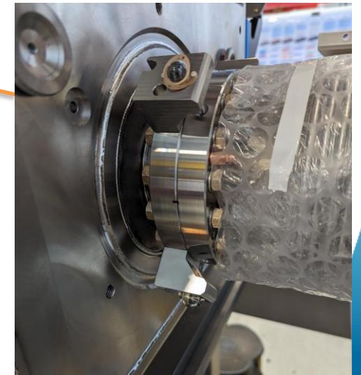
FSI target on the flange of Helium TANK of the cavities
