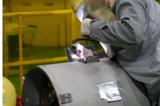
Welding of alignment markers
