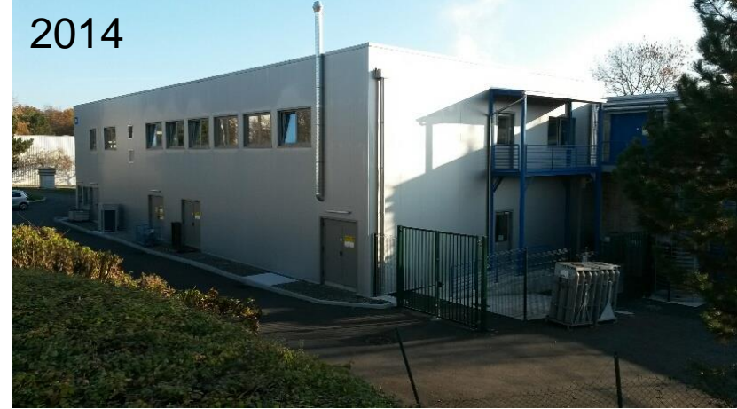
User and Operations facility building
