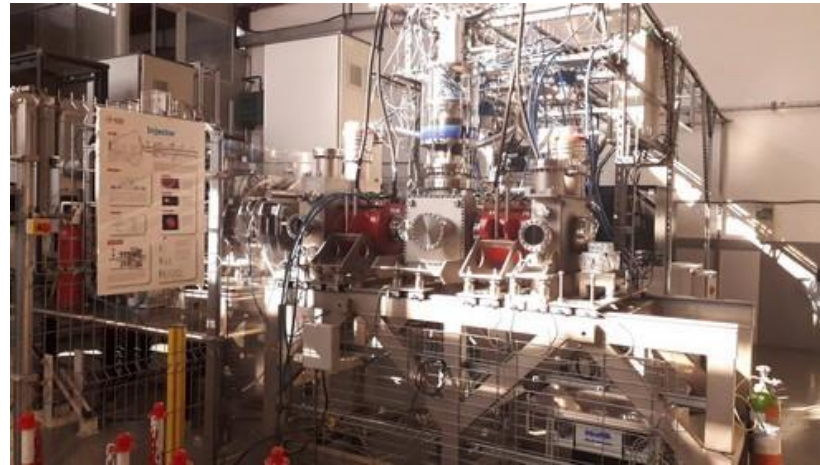
ESS-Bilbao ion source + LEPT
