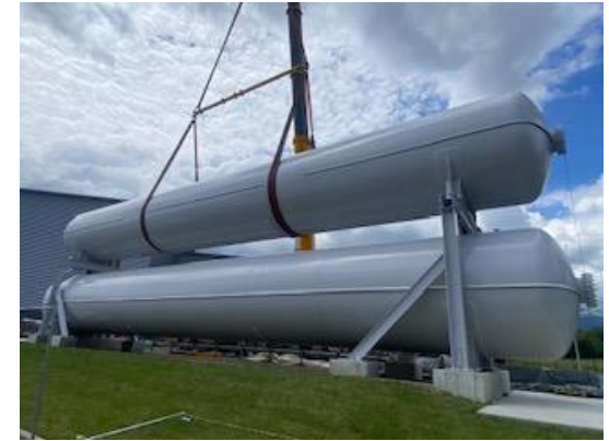
Installation of gaseous storage tank
