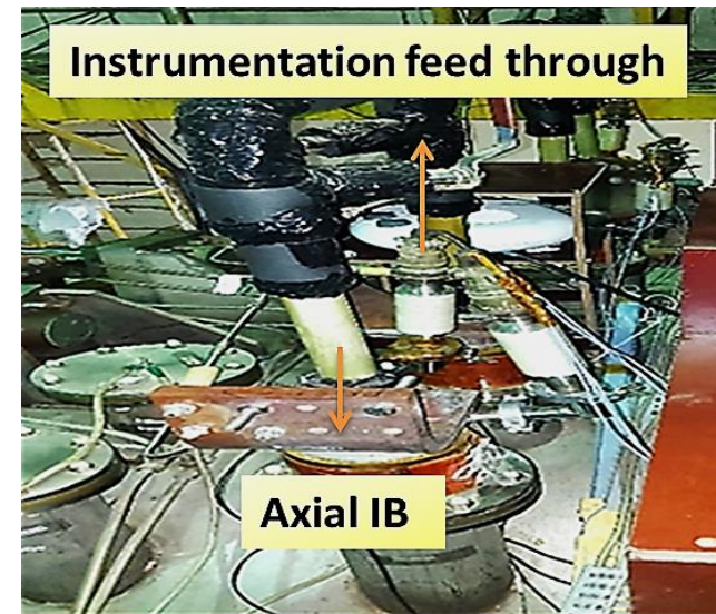
10 kA current lead outlet
