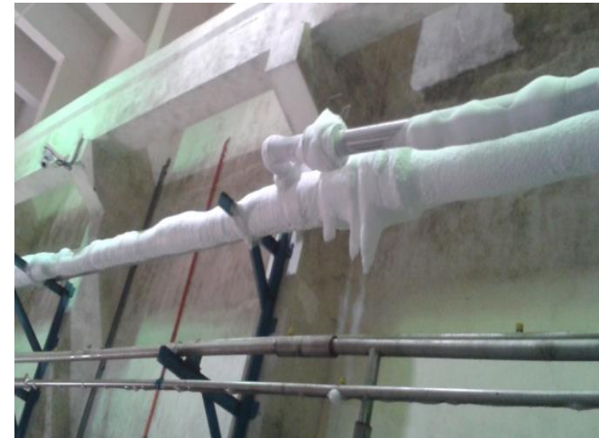
Frosting ,condensation and leakages in 80 K system
