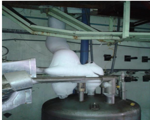
Frosting ,condensation and leakages in 80 K system
