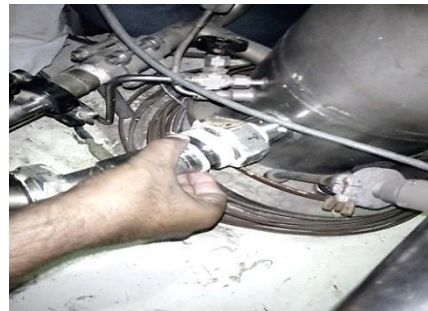
High pressure cryo grade thread sealant used in Helium connectors, Rupture disc coupler
