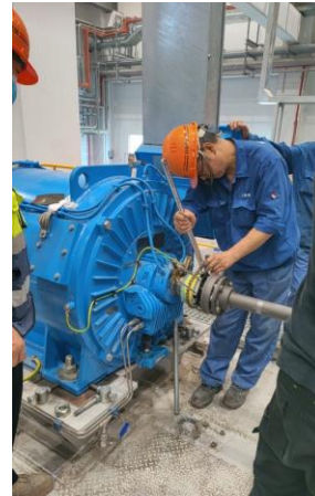
Aligning of compressor & installation coupling
