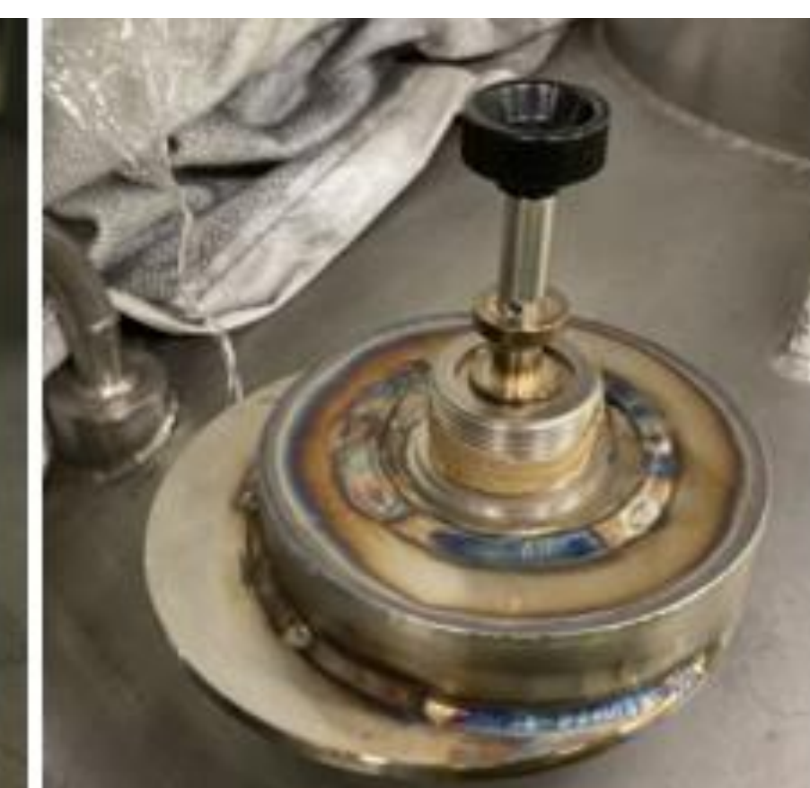
Valve top was rewelded and checked straightness by caliper gauge
