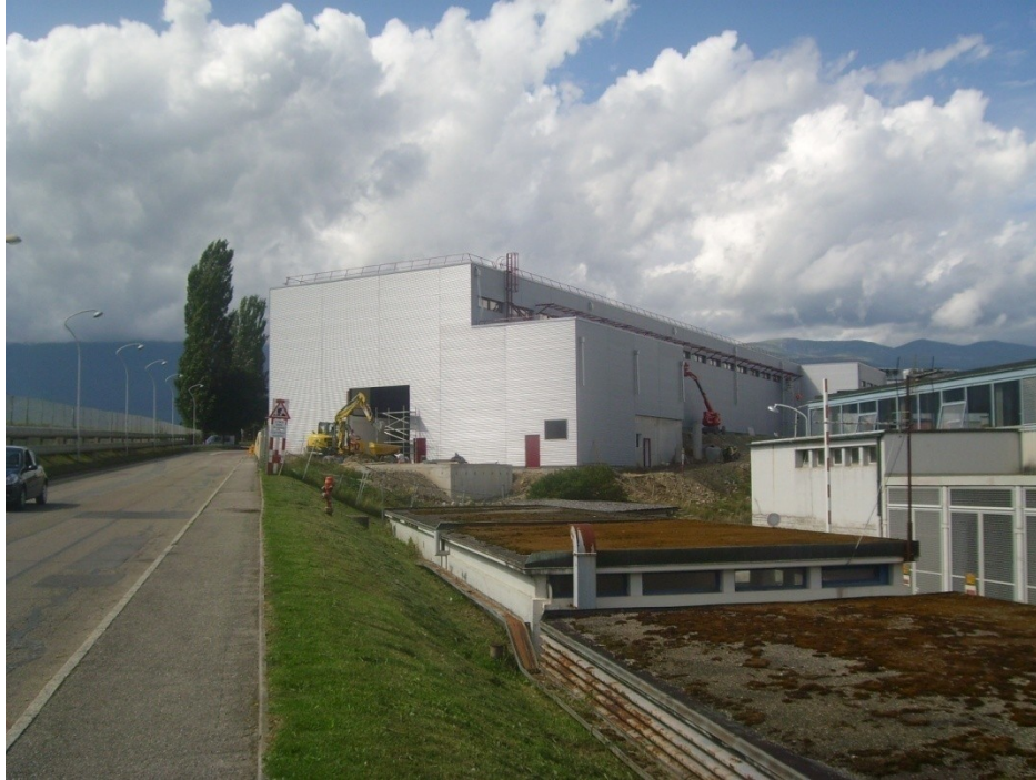
Surface building, August 2010
