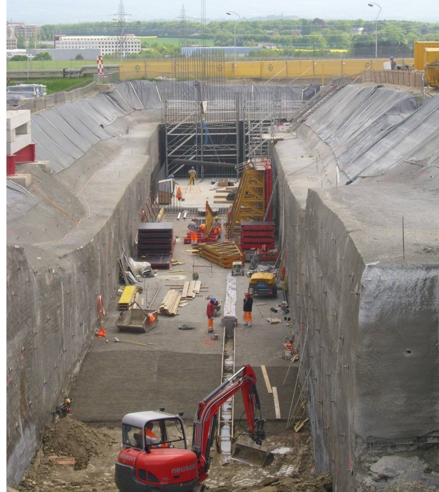
Excavation work, April 2009
