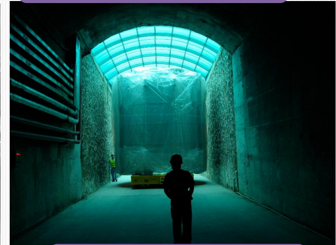
AD1 moved to hall 1
