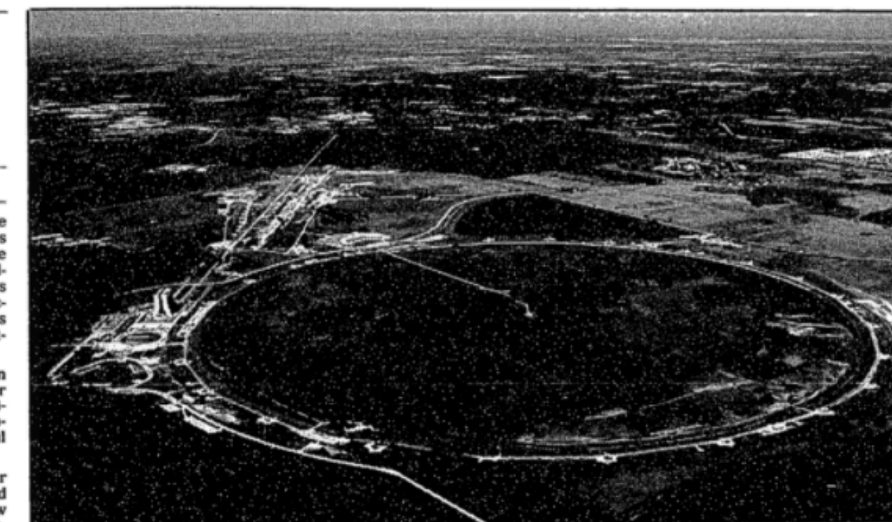
Aerial view of Fermi National Accelerator Laboratory in Batavia, Illinois, showing circular main accelerator.
