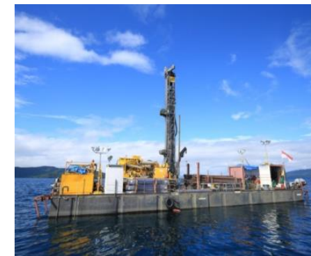
Drilling works on the lake
