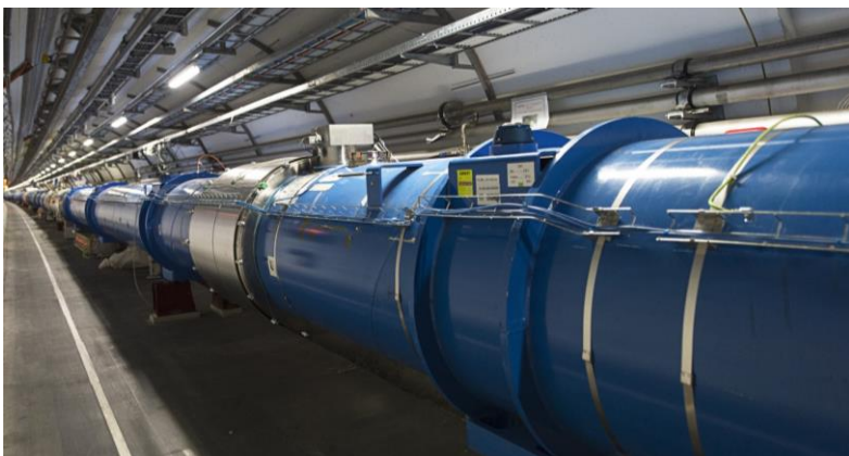
LHC dipoles (8 T) in the tunnel
