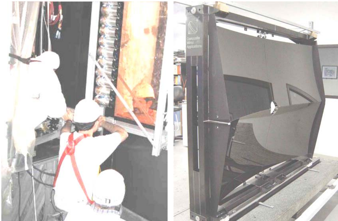
RICH-2 HPD column installation RICH-1 four uncoated spherical mirrors
