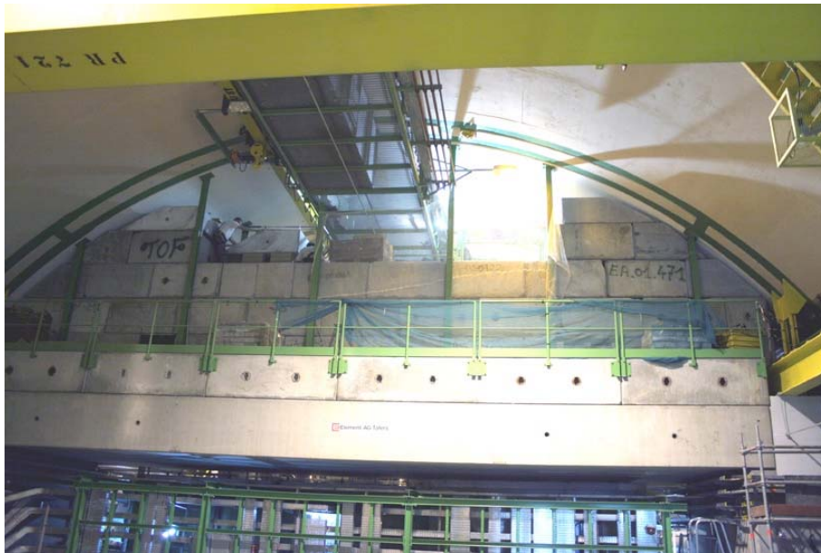
The upper part of the shielding wall
